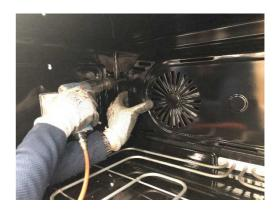
Remove the fan protection sheet by removing the screws with the help of a screwdriver.
