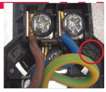
Left L1: Phase Connection Brown Cable Right NL2: Neutral Connection Blue Cable Bottom Centre: Earthing Connection Yellow-Green Cable
