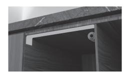
Align the supplied moisture protection tape to the cabinetry as shown. Ensure this area is free of debris before carefully applying the tape to the surface.
