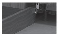
Mark the pilot hole locations for each bracket. Measure the centre of the panel and mark 237mm to each side. To determine the height of the brackets, measure the height of the lowest bracket hole against the toe kick panel.
